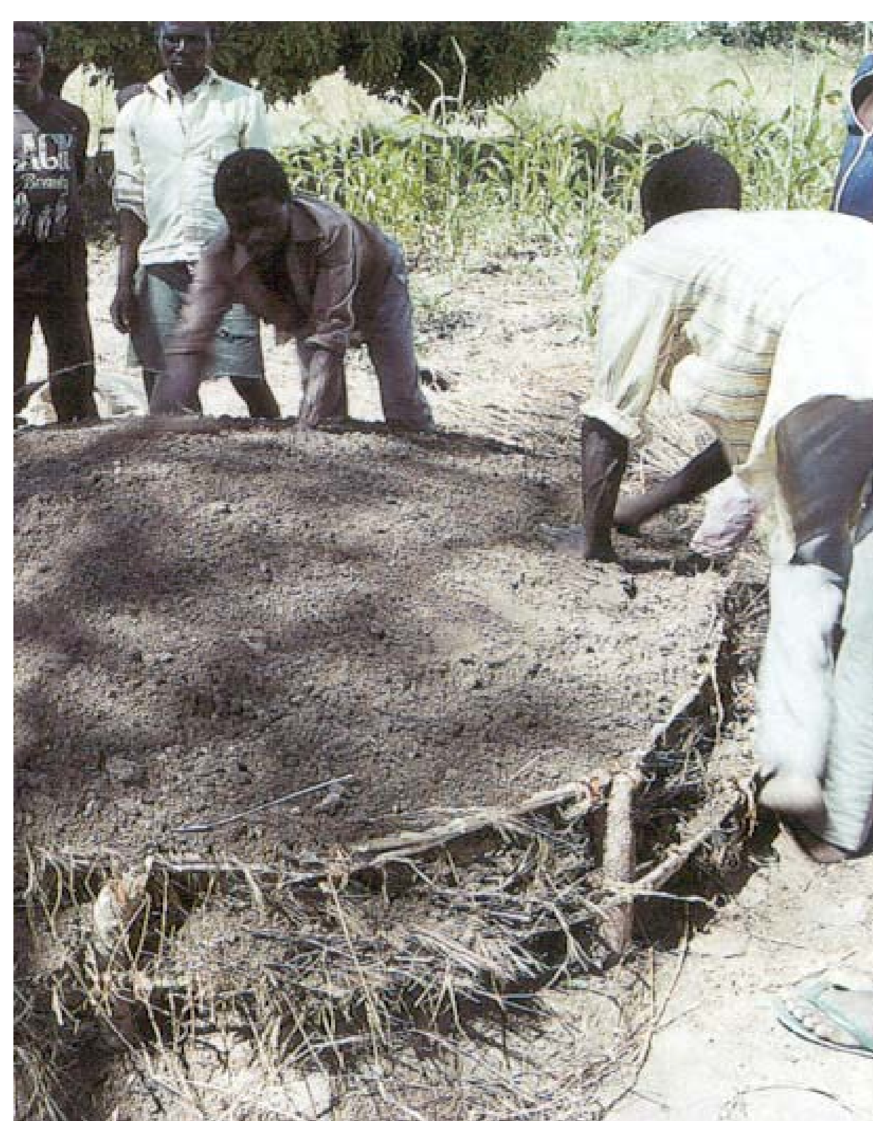
CONSTRUCTION OF THE CLAMP
